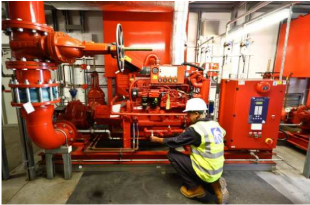
Diesel Fire Pump within Pre-Packaged Kingspan Pumphouse
