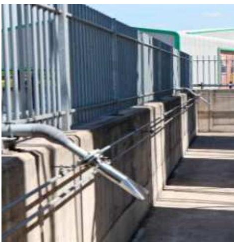
Medium Velocity water spray deluge systems to flammable liquid storage vessels
