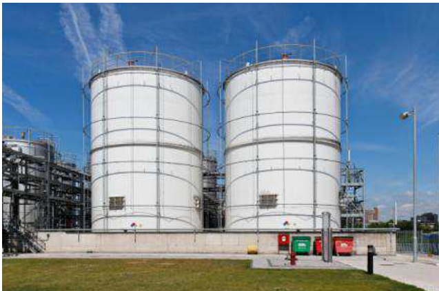
Medium Velocity water spray deluge systems to flammable liquid storage vessels
