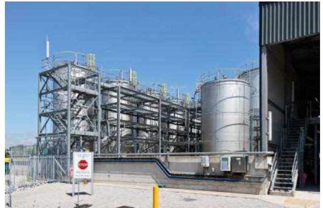
Medium Velocity water spray deluge systems to flammable liquid storage vessels
